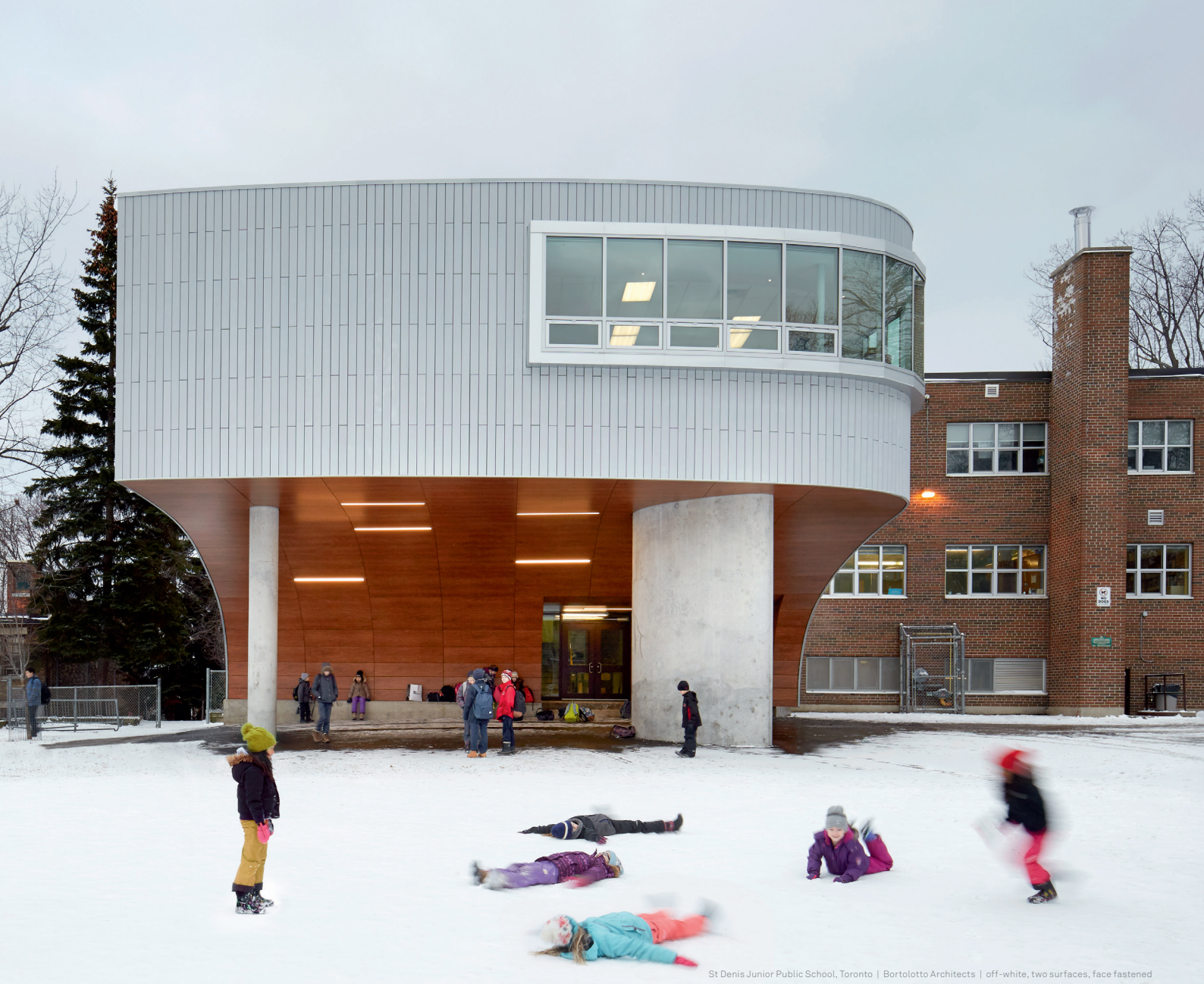
St Denis Junior Public School, Toronto | Bortolotto Architects | off-white, two surfaces, face fastened
