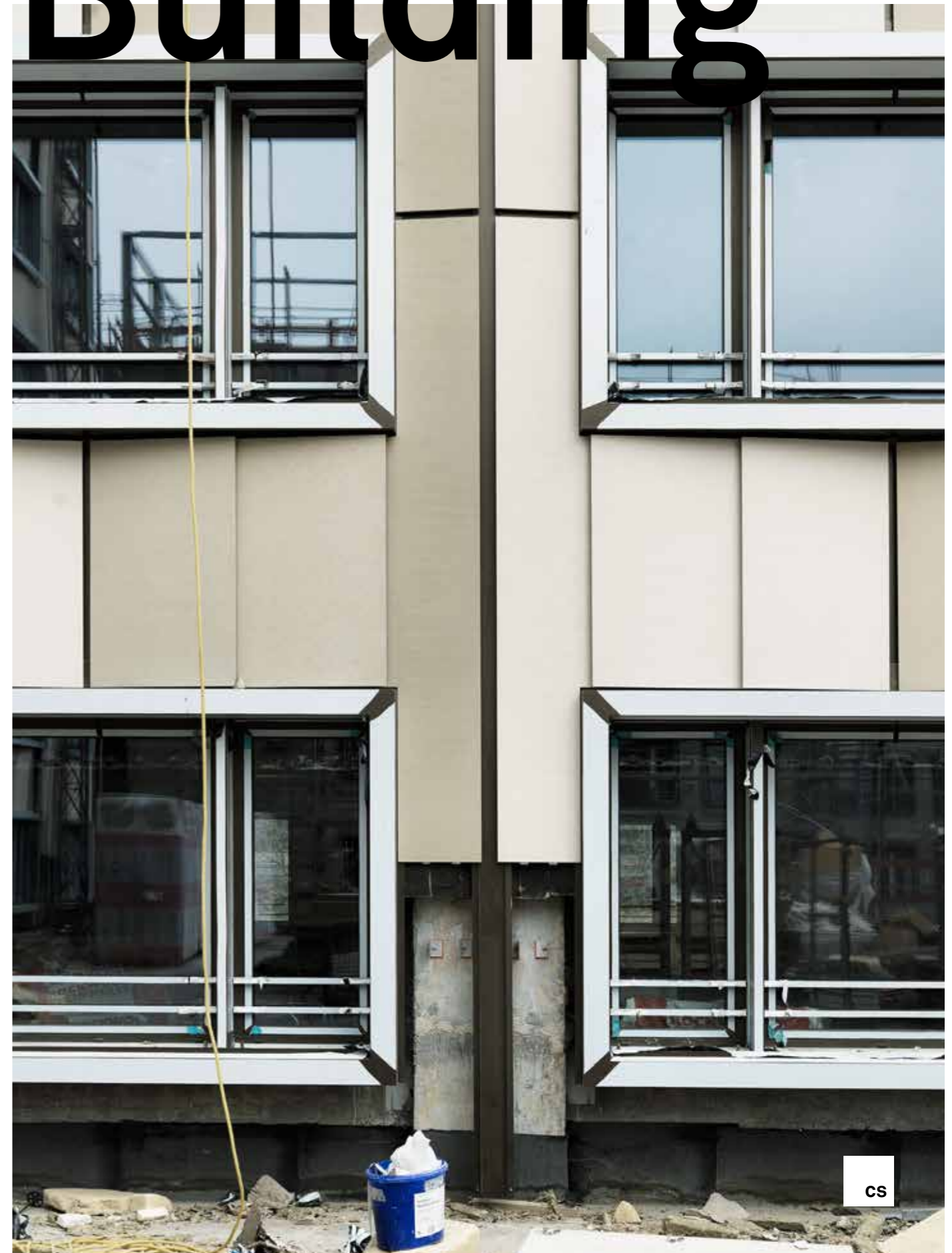
BayWa Tower, Munich, Germany | Hild and K Architects
