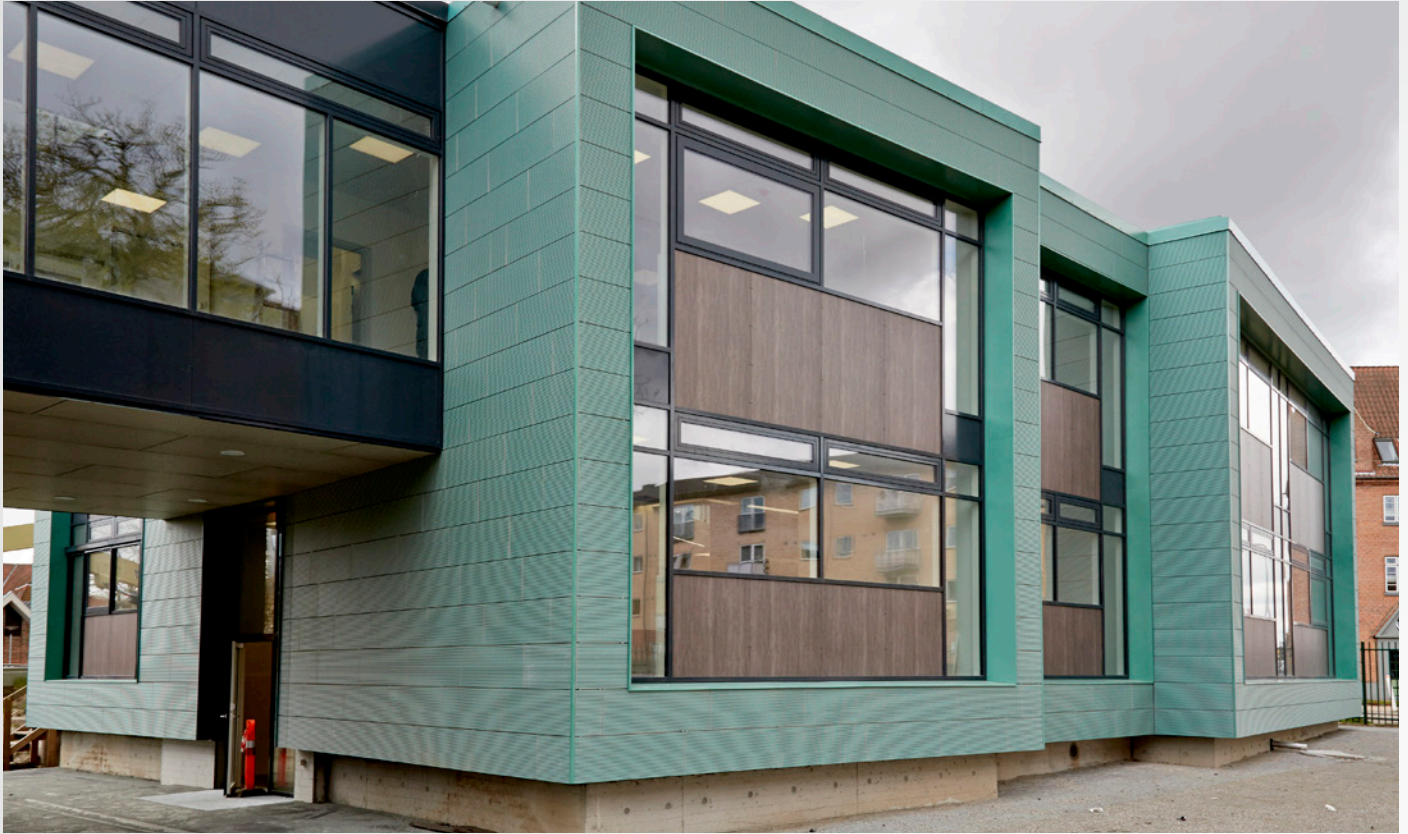
tempio® [projects] Odense Vandcenter. Denmark
